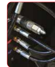
Nitrogen pressure test
